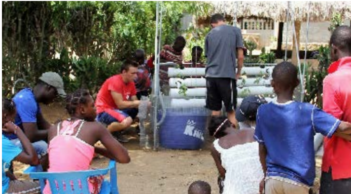
The team from Connecticut installing a new system
